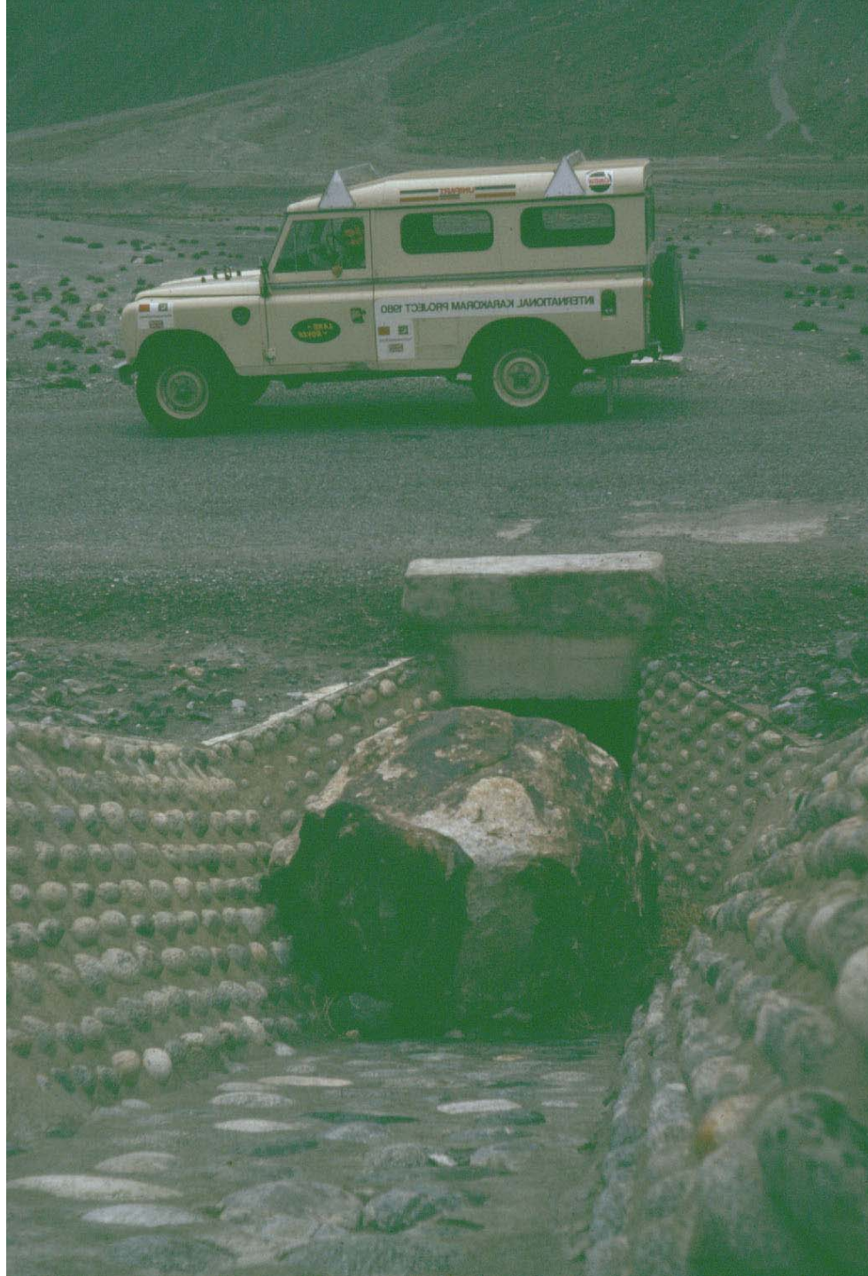
Culvert and boulder
