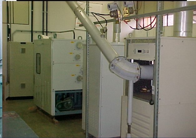
Gas microturbines and chiller
