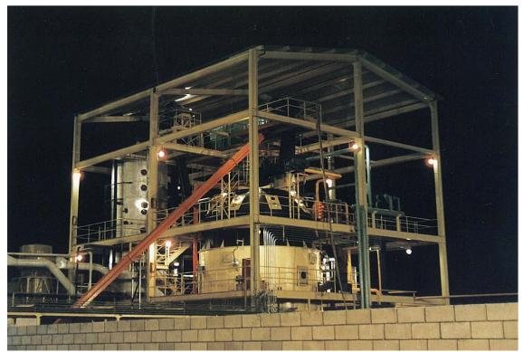
Figure 17—Typical Solvent Extraction Operation with a Deep Bed Extractor
