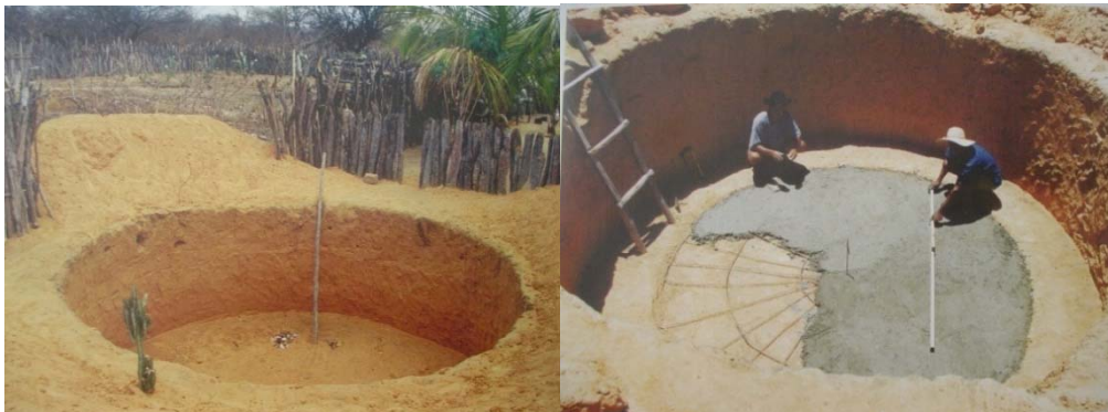
Figure 1 – Excavation of the opening and execution of the concrete flooring of the cistern
