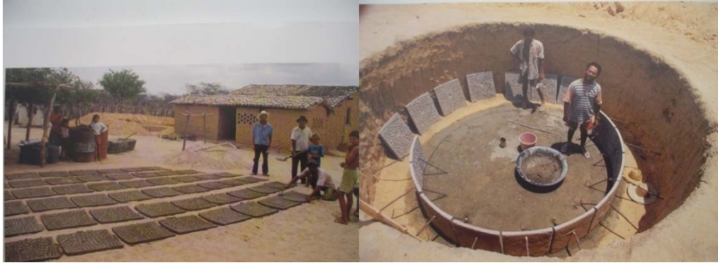
Figure 2 – Fabrication of the plaques and assembly of cistern walls
