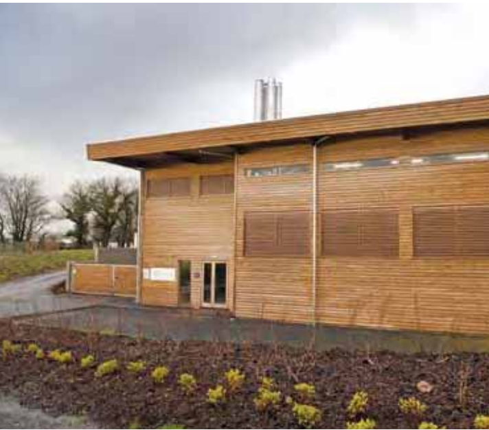
The biomass heating plant at Bluestone holiday park Pembrokeshire, Wales
