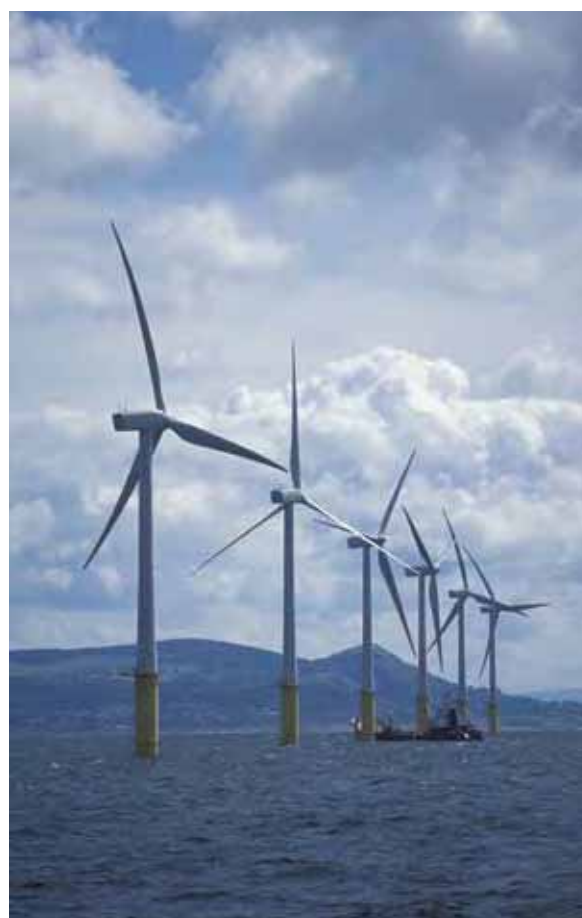
Offshore wind farms will be part of the future electricity supply
