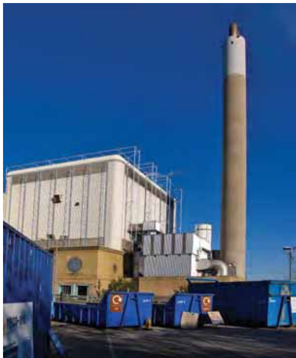
CHP facility in Lewisham, South East London Businesses are exempted from climate change Levy for good-quality combined heat and power plant
