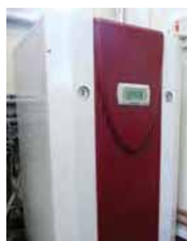
A ground source heat pump installed in a home in Wales
