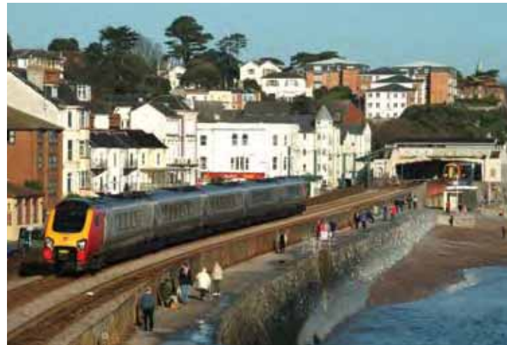
The Government is planning ahead to ensure our strategic transport infrastructure can cope with the climate change we expect will occur in the UK
