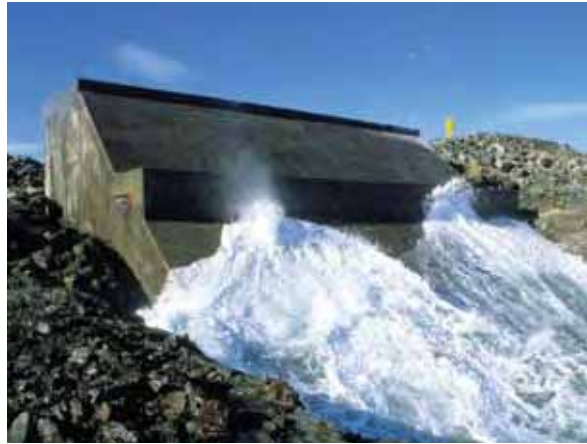
Wave striking Limpet 500, the world's first commercial-scale wave power station. Limpet generates 500 kilowatts of electricity, enough to power 300 homes (Islay, Scotland)
