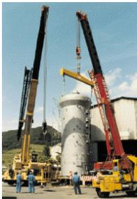
The Desolventizer-Toaster (DT) serves the purpose of removing the solvent from the meal, which can be directly used as an ingredient in animal feed compounds.
