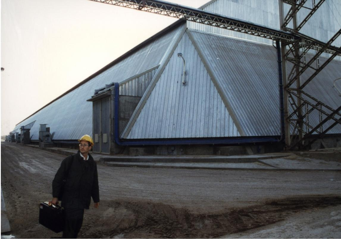
**Top Section of Underground Soybean Storage Structure**
